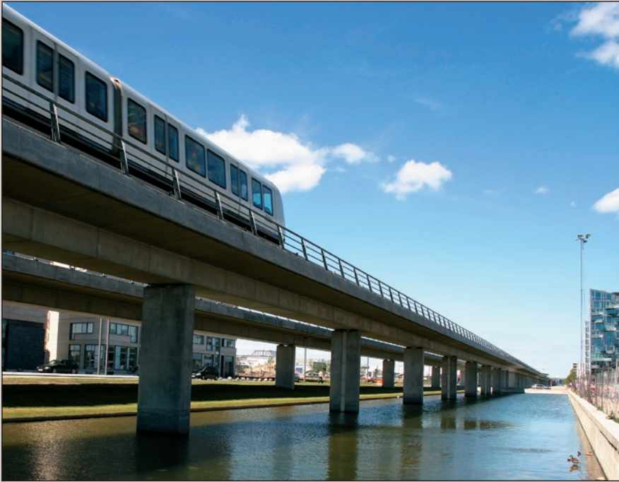
The Metro is the backbone of transport in Ørestad, running every 5 minutes. It is elevated, to make it visible and to minimize impact at ground level. Photo: Lene Skytthe/By og Havn.
